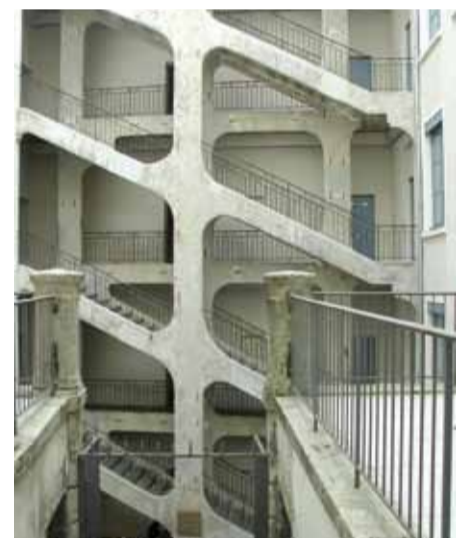
Cour des Voraces, passageway across the slopes of Croix-Rousse – famous for its monumental, open-plan staircase, constructed in 1840, Canut style. Sheltered the Canuts during their revolts, site of the 1849 battle, photograph, 20 th c.
